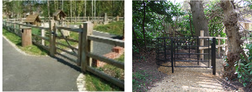
Examples of typical accessible barriers
