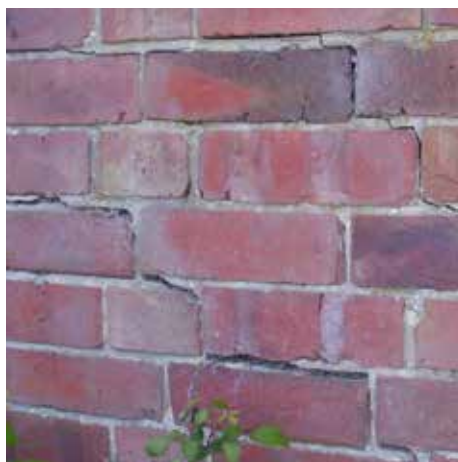
Failed pointing in brick walls can allow driving rain to penetrate
