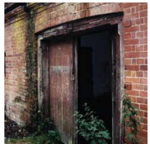
The guttering to this building is cracked in various areas. The result is severe moisture damage, dampness within the building and erosion of the brickwork
