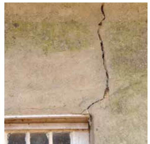
Lack of general maintenance can lead to a break down of the fabric allowing ingress of moisture
