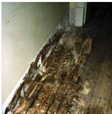
This outbreak of dry rot developed as a consequence of no through ventilation in the floor void
