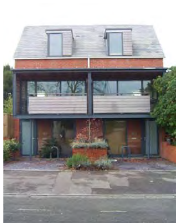
A pair of modern semis picking up the street rhythm where an accessible space for waste storage, meters and ancillary storage has been 'designed' as part of the balanced street façade.
