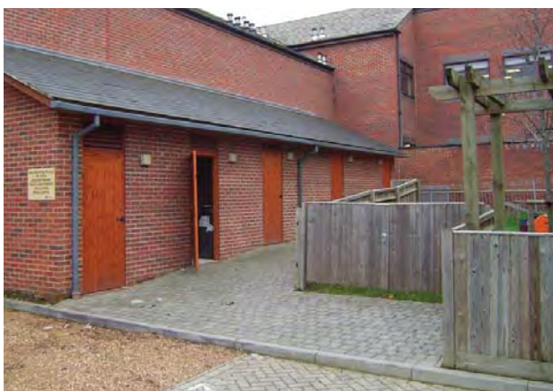
A series of enclosed waste stores for a multiple flat development have been built against an otherwise blank wall. The enclosing structure picks up reference particularly in terms of materials from the main development.
