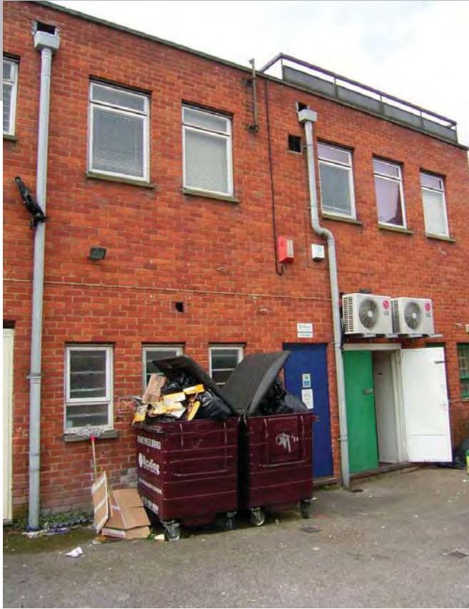
This illustrates the inevitable problems of unsightly accumulation of waste where no area is specifically allocated to bins.
