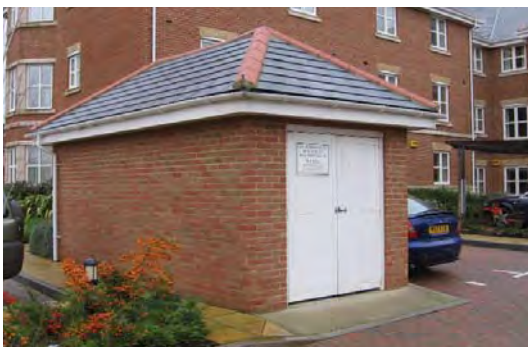
Here a waste storage building has been designed as an integral part of the development.
