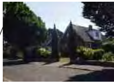
Group of matching chalet style dwellings in garden settings around an avenue of hornbeam. Low front boundaries allow the gardens to offer a very green and pleasant communal amenity.
