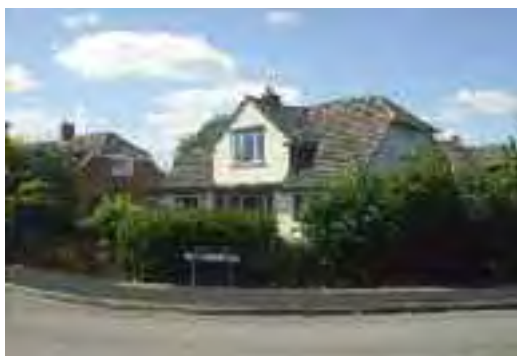
Fig 6.4 Most of the dwellings in the western half of the area were built as 1½-storey chalet bungalows exhibiting a similar form with half hipped roofs and central gable.
