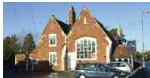
The Old School - The surrounding car park, especially its unsympathetic shrubberies is a minor detraction from the rich use of materials and intricate details of the old school building.
