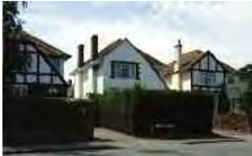
Fig 7.10 An impressive row of similarly formed villas face the entrance to Highfield Avenue.
