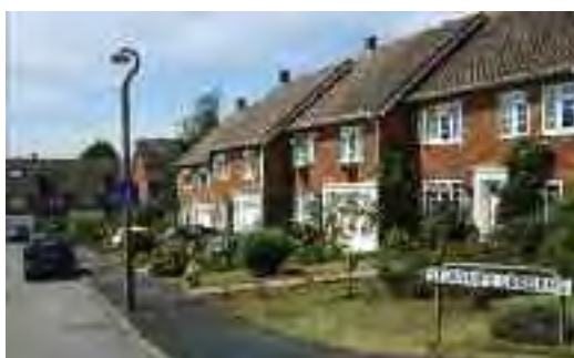
Fig 7.16 St Anne's Garden: open plan, consistent gardens and dwelling forms are important. Roof planes uninterrupted by dormers, and gardens retained forming a predominantly green landscape are strong characteristics of the place.
