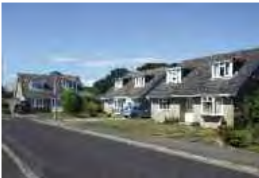
Fig 9.7 Open plan bungalows and chalet bungalows are typical of Harford Close.
