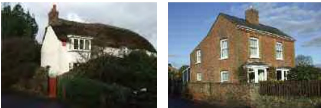
Fig 8.1 North Street cottages.
